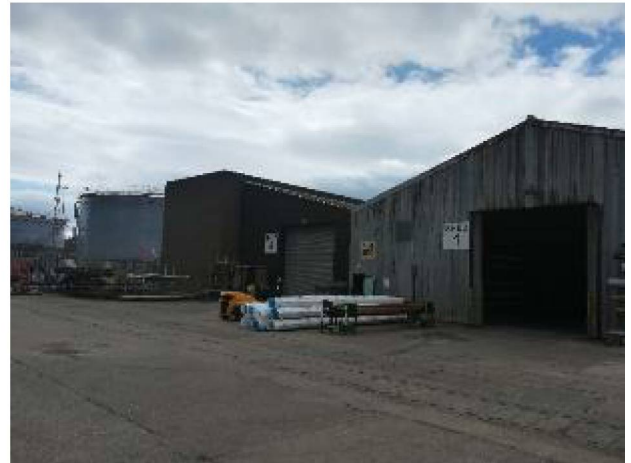
Photo E-12 - Steel-framed and steel-clad buildings within the Site
